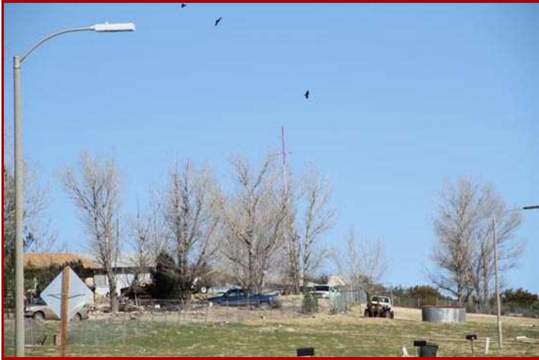
Fig. 1 Shu'luuk Wind Meteorological Tower, on Kumeyaay Road, Campo Indian Reservation, San Diego County, California (February 12, 2013).
